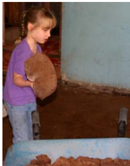
Brittany pitching in with new floor at Casa de Niños.
